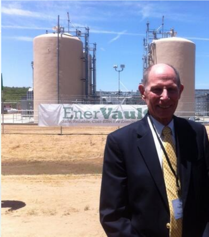
Dr. Lawrence Thaller Father of redox flow battery In front of a 250-MWh FeCr system by EnerVault
