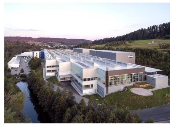
Headquarter J.Schmalz GmbH Glatten, Germany
